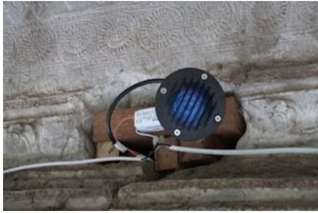
SokAn renovated Angkor Wat with the light by craving it.
