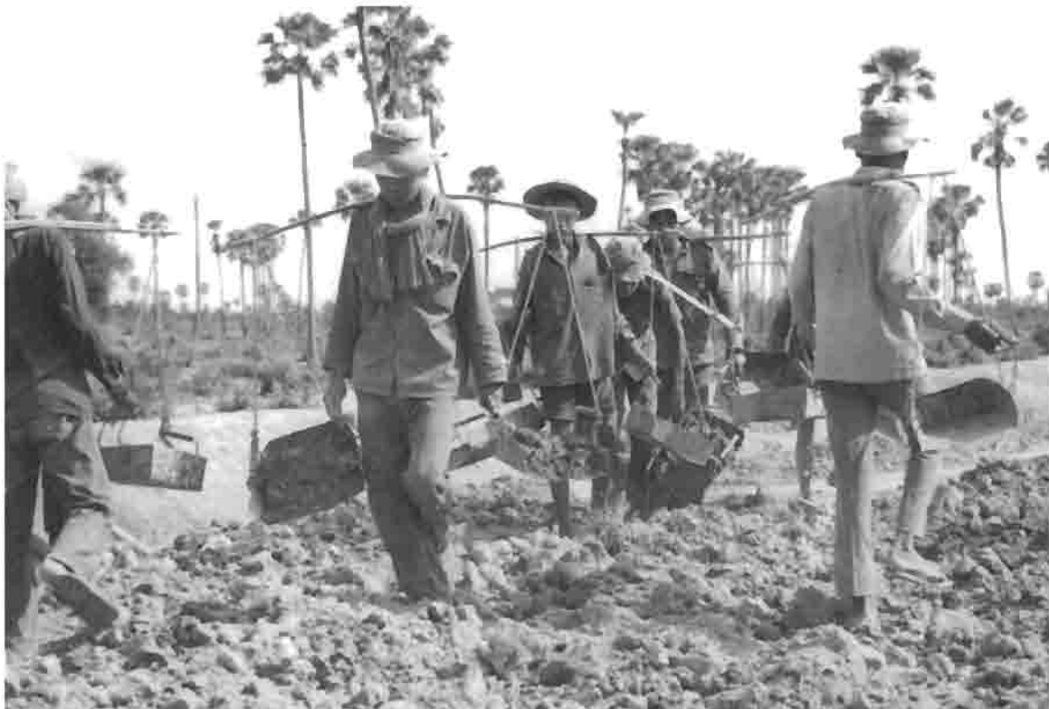
Transporting dirt on an irrigation project. (Documentation Center of Cambodia Archives)
